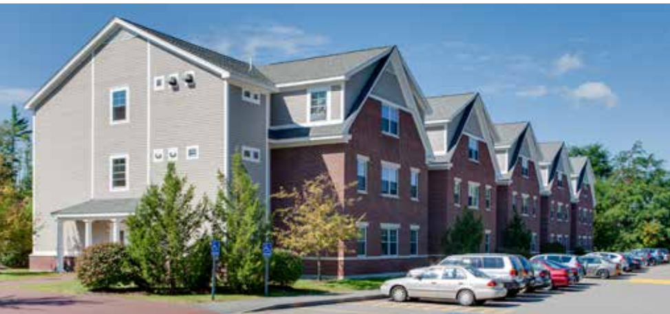
The school's 2006 dormitories were retrofitted with new pumps for more efficient operation.
